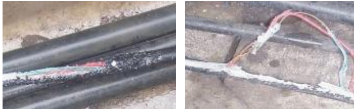
PHOTOGRAPHS COURTESY OF HORSHAM AREA RESIGNALLING THAMESLINK 2000
