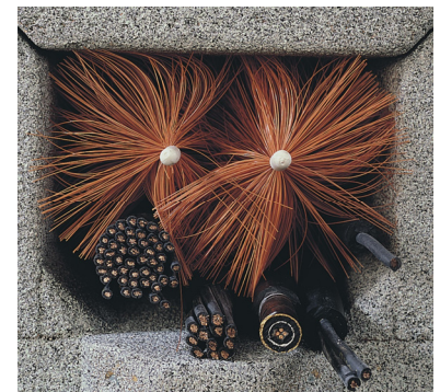
RODENTBRUSH FITTED TO TRACKSIDE TRUNKING
